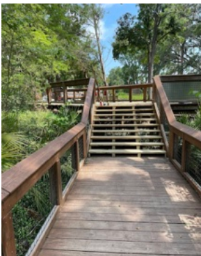
The new stairs and walkway at Madison Blue State Park. Photo by Fred Stratton.
